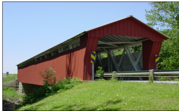
McColly Covered Bridge 13-1.56 over the Great Miami River
